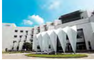
Tainan Plant (Diamond-rated Green Building)
